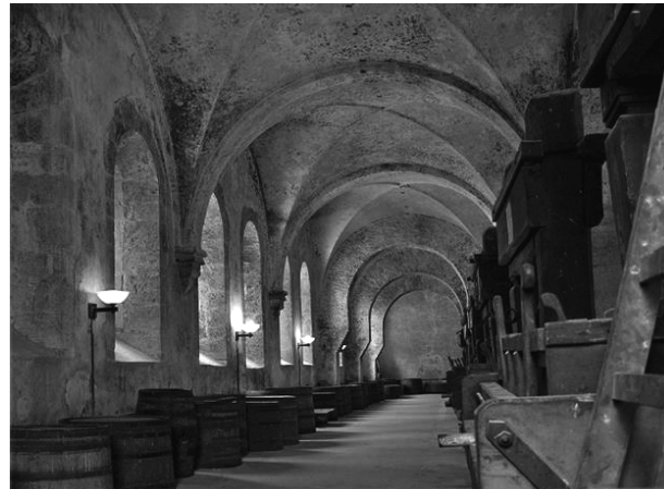
Figure 18: Old wine cellar with original wine presses from the Middle Ages (still functional). Source: Stadt Elteville ©
