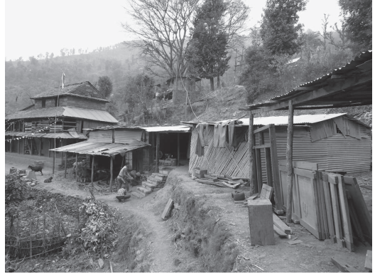
Photo 2 : Light Damaged house (left), animal shed (central: back of a man) and temporary hut (right) in Dhungagadhe (Feb. 2016)
