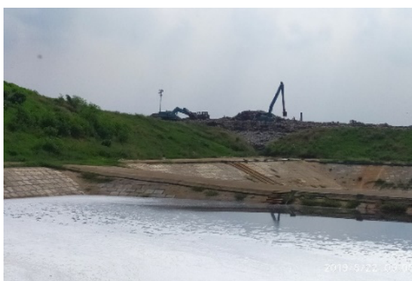
DNCC landfill site, leachate treatment pond (Amin Bazar)
