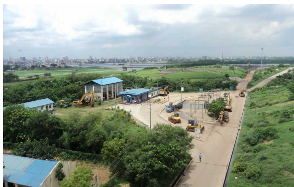
DSCC landfill site, control building with weighbridge and car wash facility (Matuail)
