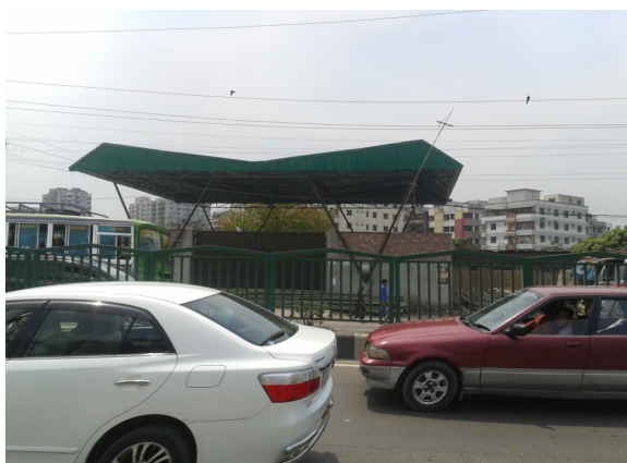
Waste transfer station, DNCC
