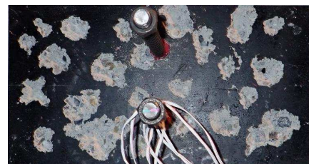
After setting the anchor bolts
