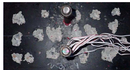
After setting the anchor bolts
