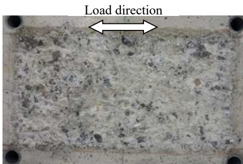
Photo 4-5 Failure status of CH-M100LM-cy
