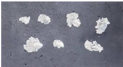
Before setting the anchor bolts
