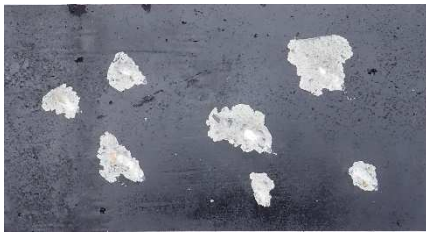
Before setting the anchor bolts
