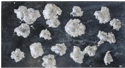
Before setting the anchor bolts
