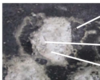
Photo 4-4 Failure mode of single roughened part
