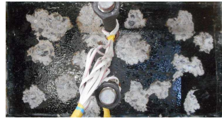
After setting the anchor bolts
