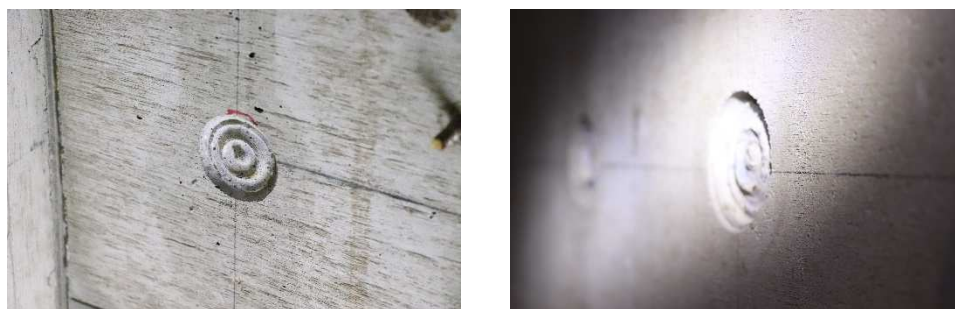
Photo A1-4 Cylindrical shear-key
