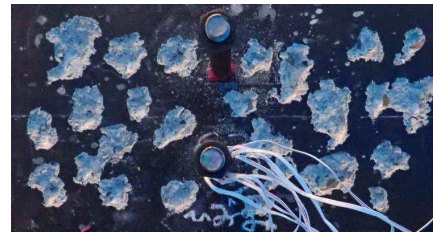
After setting the anchor bolts
