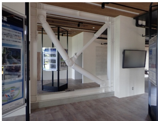
Photo 1-1 Seismic retrofitting by damping brace
