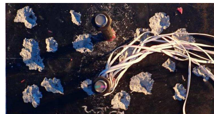
After setting the anchor bolt
